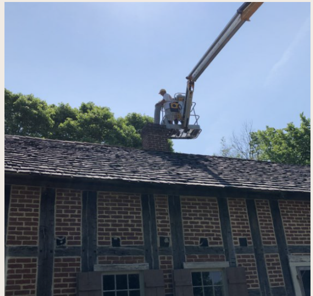
New Chimney sleeve is installed using a 60 foot manlift!
