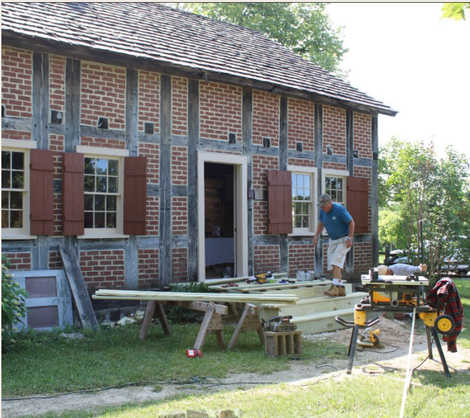
New steps and porch under construction
